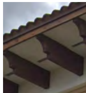
9 WOOD OUTRIGGERS BROWN TEAK WOOD REF. MATCH EXISTING SHIPPING CENTER REF. COLOR CUSTOM BROWN SEE 3/A-400
