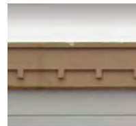
13 DETAILED BANDING SMOOTH STUCOCO FINISH REF. MATCH EXISTING SHOPPING CENTER COLOR CUSTOM TAN SEE 2.2/A-400
