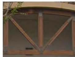
10 WOOD ARCHWAY BROWN TEAK WOOD REF. MATCH EXISTING SHIPPING CENTER REF. COLOR CUSTOM BROWN SEE 3/A-400
