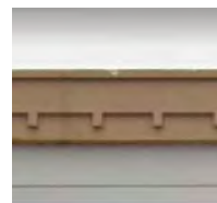
13 DETAILED BANDING SMOOTH STUCOCO FINISH : REF. MATCH EXISTING SHOPPING CENTER COLOR CUSTOM TAN SEE 2.2/A-400
